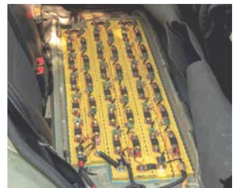
Large and/or unattended battery storage areas
